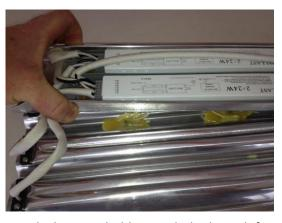
12. Push clear LED holder into hole through front of reflector.
